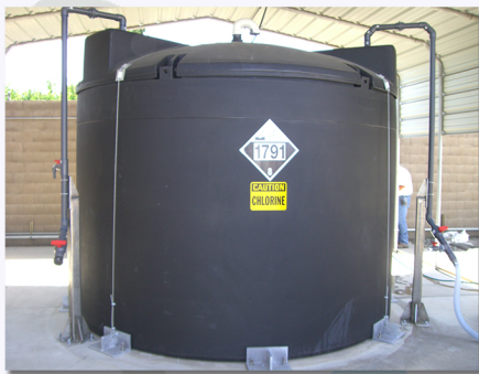
SAFE-Tank® Fully Contained Double Wall Tank Systems
