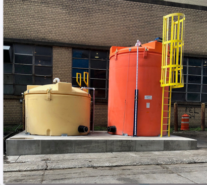
SAFE-Tank® Fully Contained Double Wall Tank Systems
