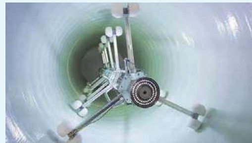
UV Mainline Lining
