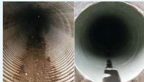
Before and After Spincast Lining
