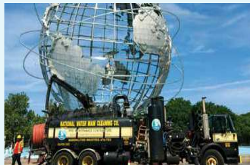
CCTV-Sewer Cleaning-Catch Basin Cleaning
